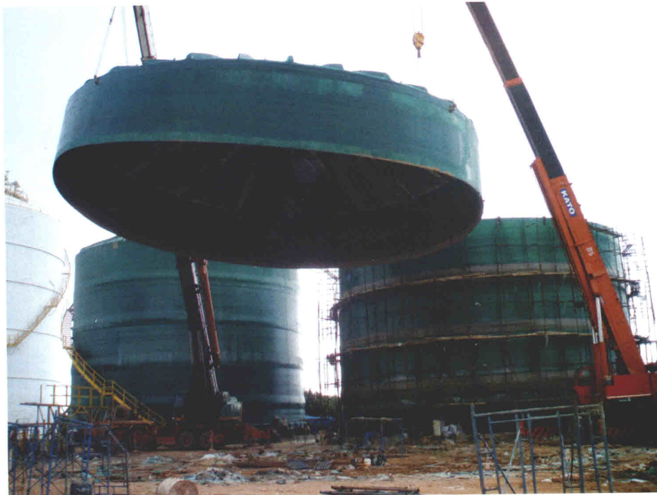
The top can and dish assembly being lifted into position.
