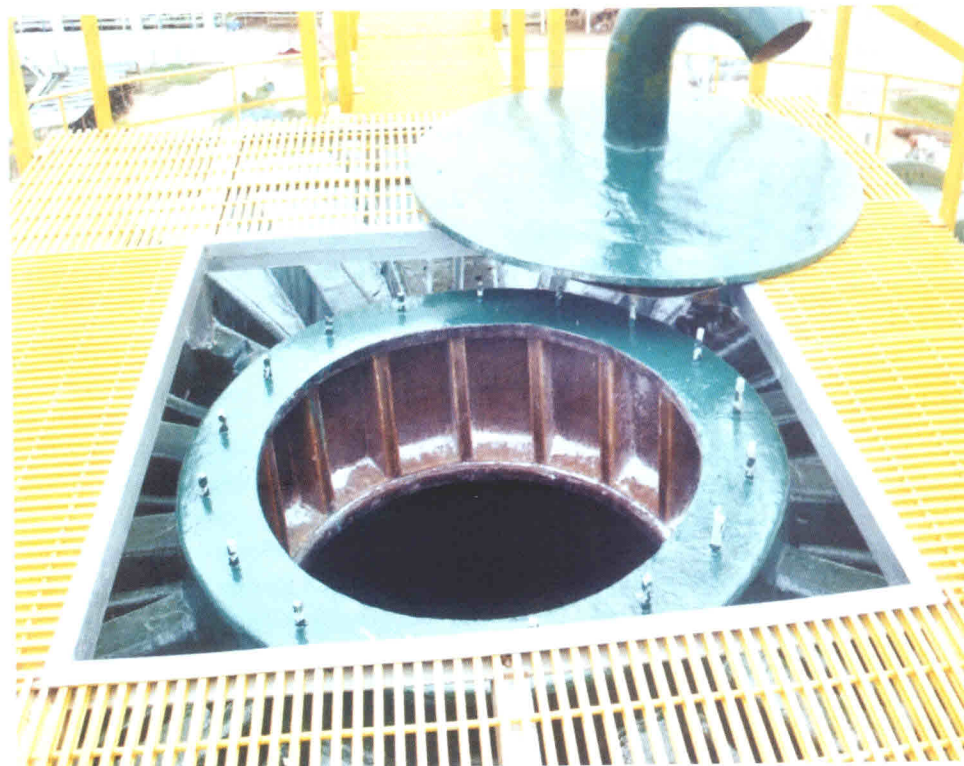
The large compression ring at the top of the dish.
